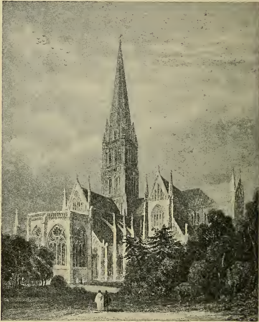
SALISBURY CATHEDRAL, from the southeast ; built, 1200-1250. The spire rises 404 feet from the ground. — From Cathedral Churches of England .
